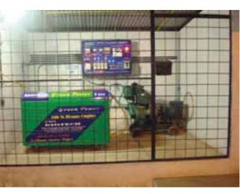
biogas scrubber, dehumidifier, control panel, power distribution system, and Exes Gas reservoir.
